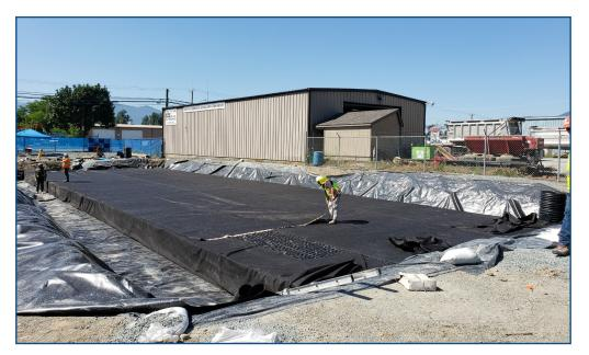
This site required increased onsite storage required by the Municipality, high water table & constant heavy traffic loading on the tank. We used the Graf EcoBloc Maxx block to create this 240 m<sup>3</sup> detention tank, complete with accessories like the manway extension in the photo below.
